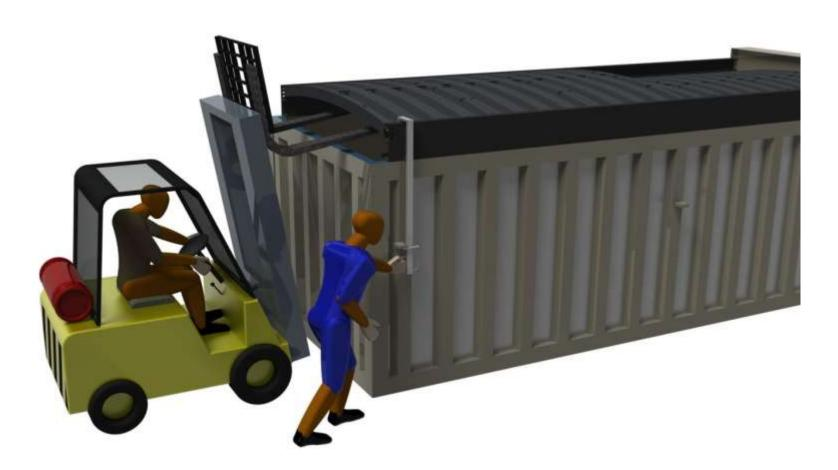
Once this lid section is fully home and secured, its time to test the lids travel freely, before the channel frame end section is fitted.
