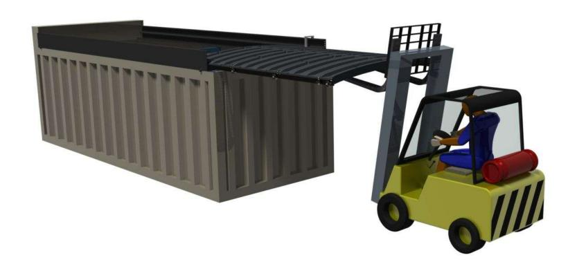
First section is then lifted carefully into the end of the container's channel assembly ideally using a fork truck with fork leg extensions.
